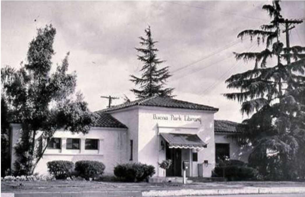
Figure 7 Second Public Library, ca. 1935 Source: Buena Park Library District Photo Historical Collection
