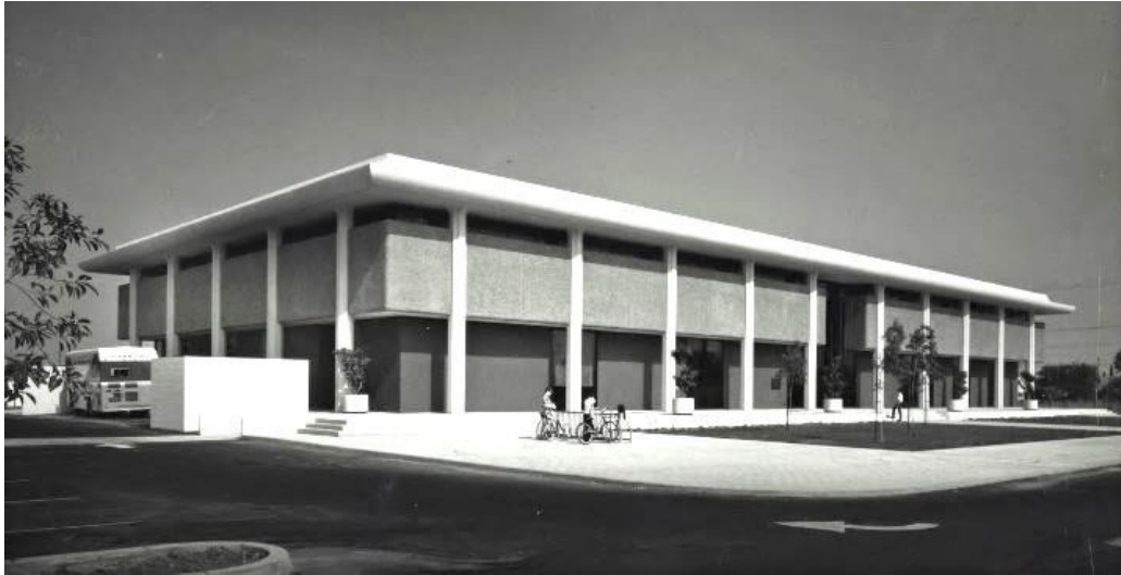
Figure 14 East Facade, right, South Facade, left, camera facing northwest
