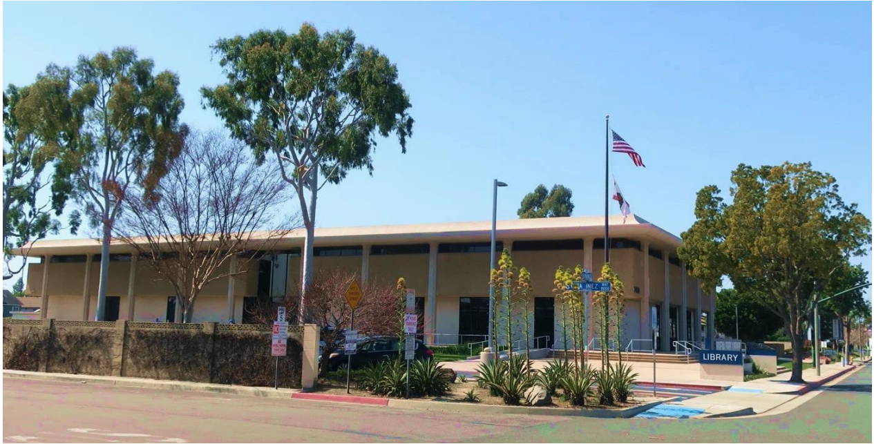
Figure 18 East (Primary) Facade SOURCE: Taylor Loudon for Lamprecht | Loudon
