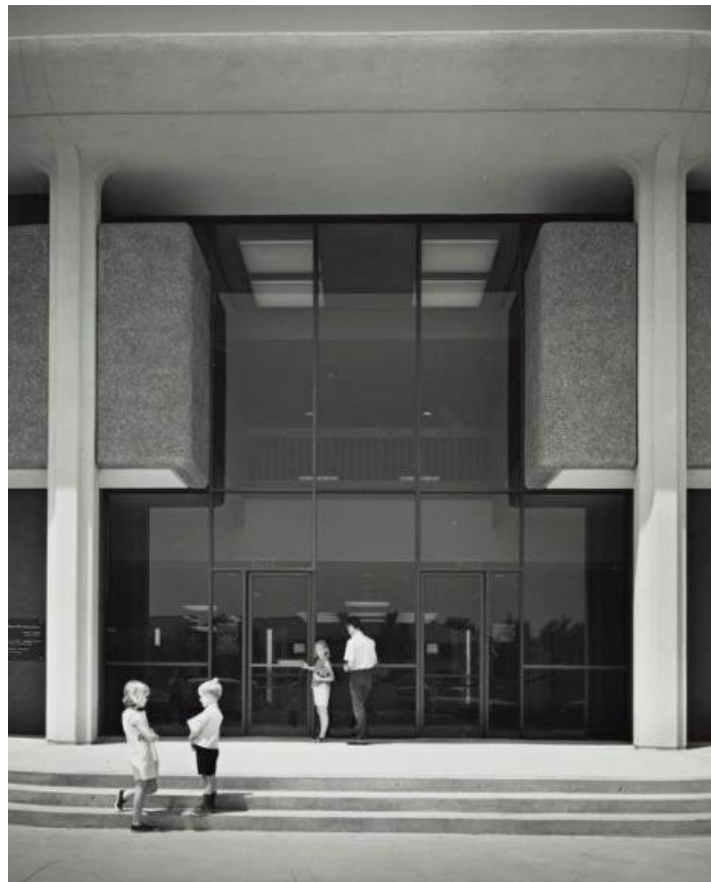
Figure 15 Primary Entrance, East Facade; camera facing west
