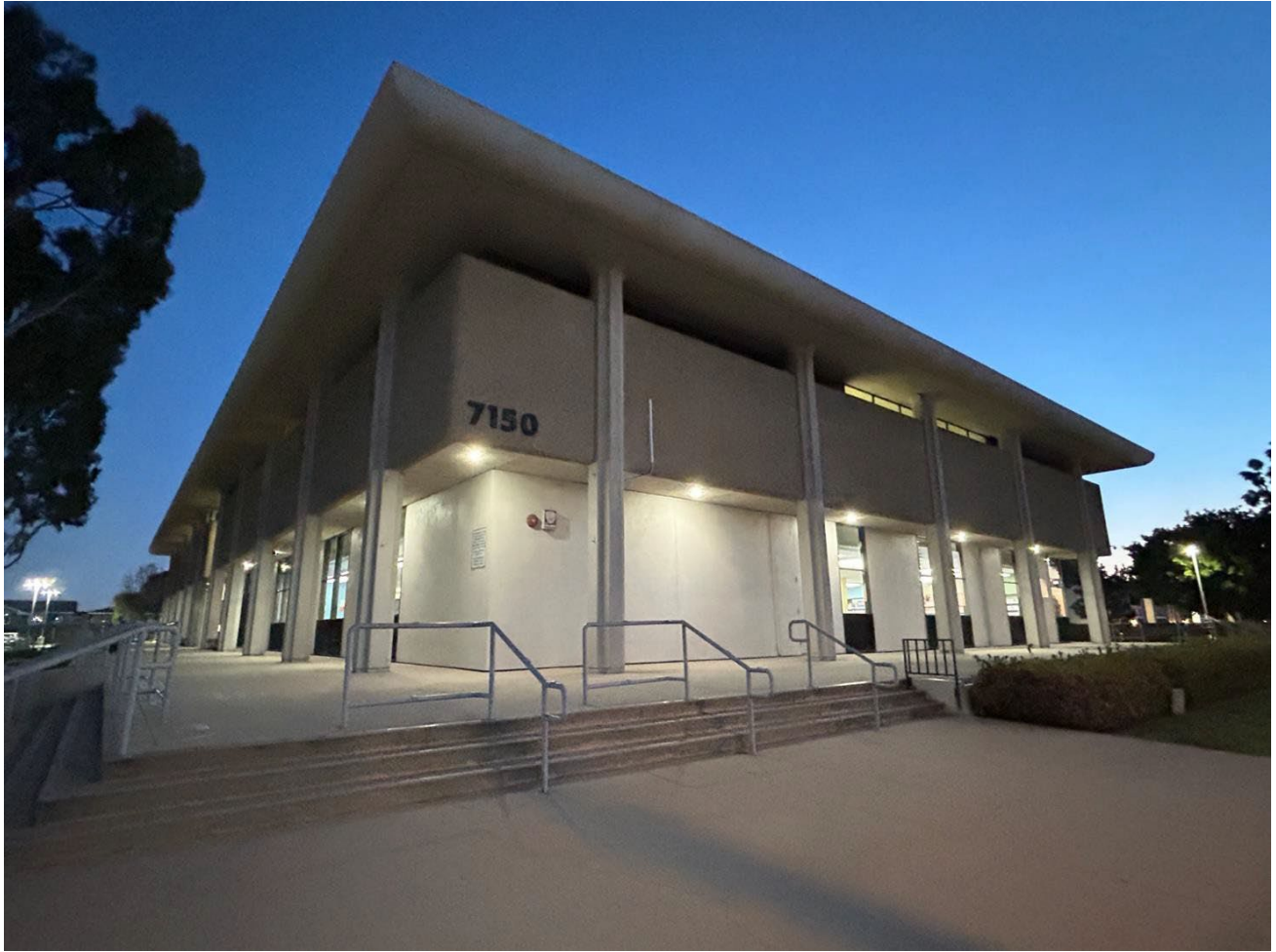
Figure 24 Library at Night, North Facade SOURCE: John English for Lamprecht / Louden
