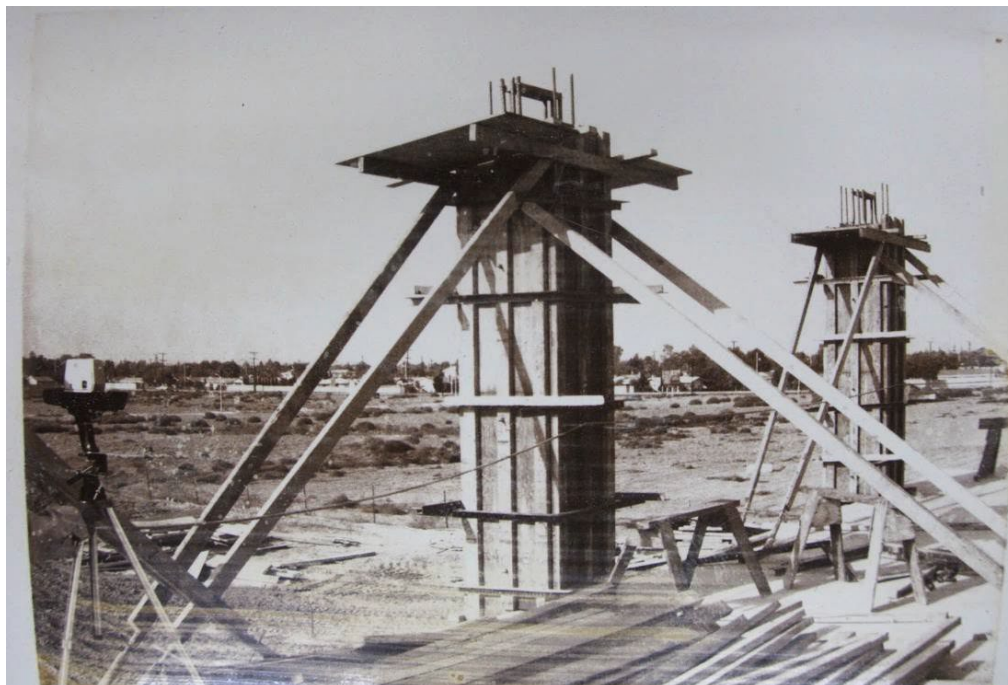
Figure 11 Constructing the Columns
